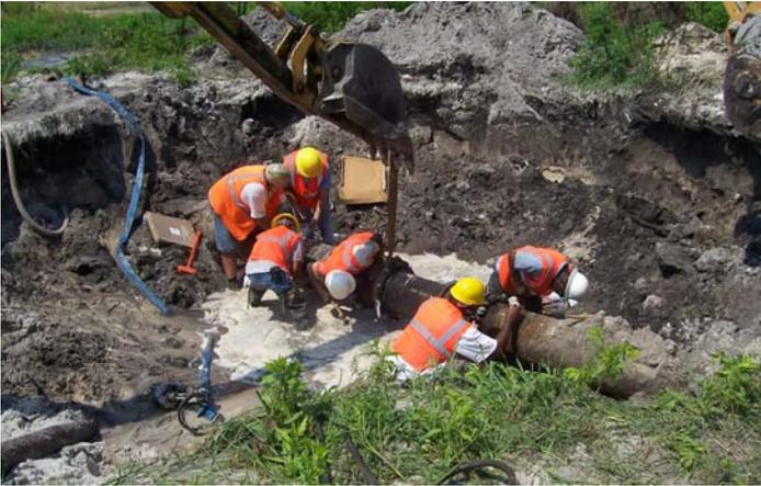
Emergency pipe repair work at the city's irrigation system for their reclaimed water.
