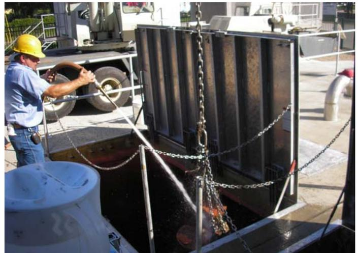
Preventive maintenance work for a pump station submersible pump.
