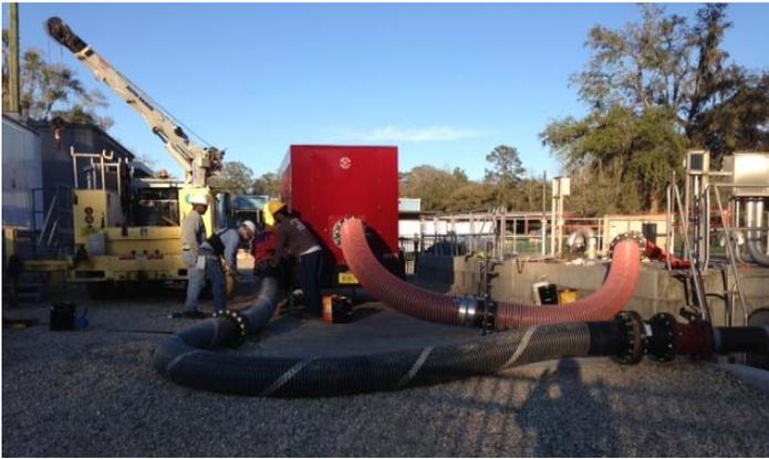
The pump station team performs a station by-pass for scheduled repairs.
